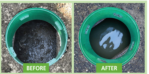
Aerobic Septic System After 4 Weeks
